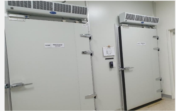
R-318, 319 Material storage
